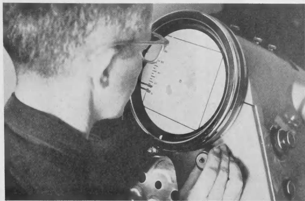
AN ESSO Research scientist examines a hydrocarbon sample on the screen of an electron microscope. The scale, right, is in microns. The electron microscope permits useful magnification up to 100,000 fold. UN CIENTISTA di Esso Research ta examina un muestra di hidrocarburo ariba pantalla di un microscope electronico. E escala, abao, ta den microns. E sorto di microscope aki ta permiti magnificacion te 100,000 vez.
